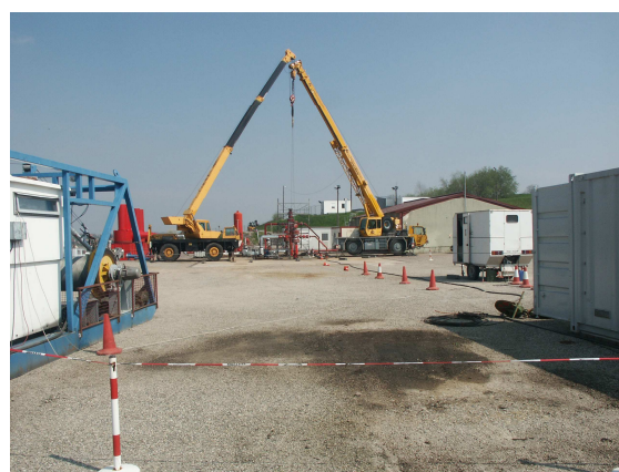
Figure 3: winches, cranes and recording unit on GPK2 platform.
